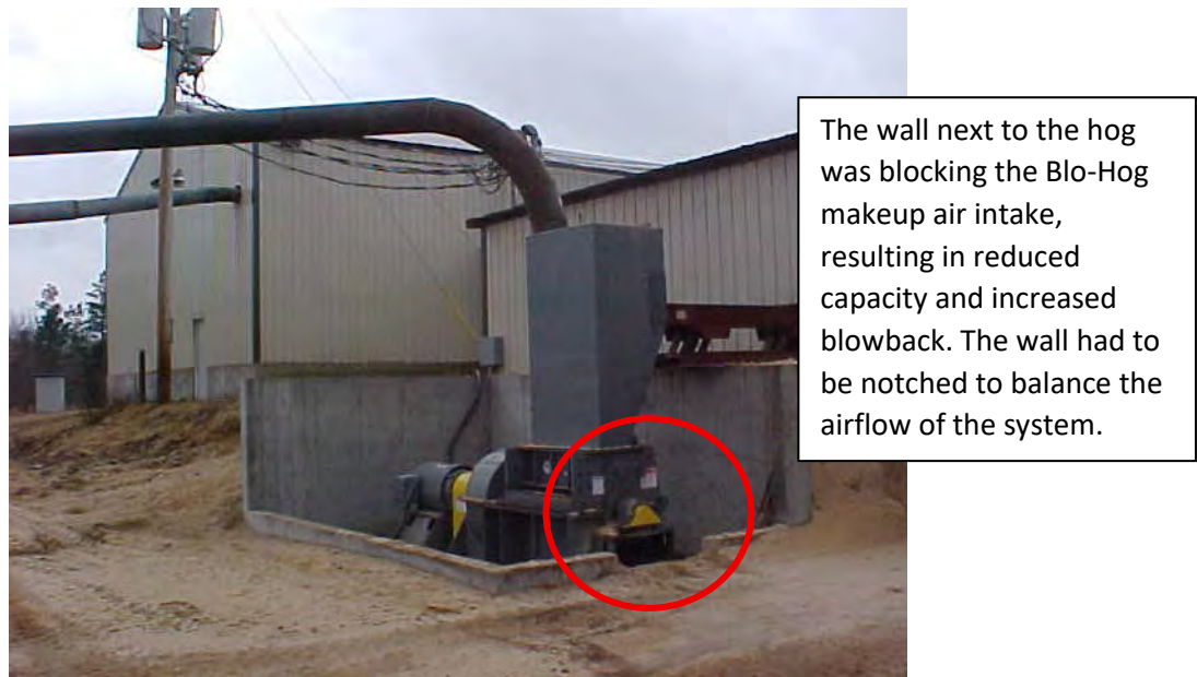
Figure 5.23: Airflow Issues from Blocked Makeup Air Inlet
