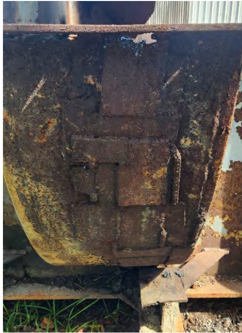
Figure 5.19: Fan Scroll Worn Beyond Repair
