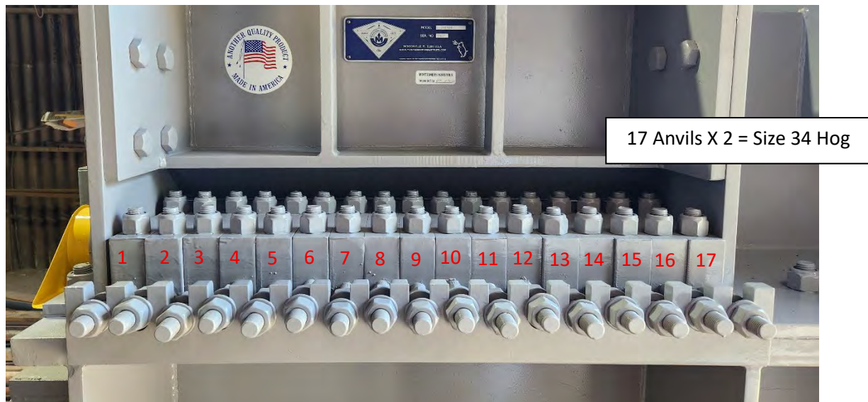
Figure 3.17: Counting Anvils to Determine Hog Size
