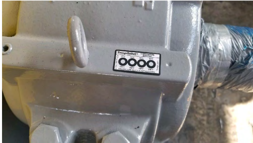
Figure 4.105: Tempilabel Temperature Monitoring Decal
