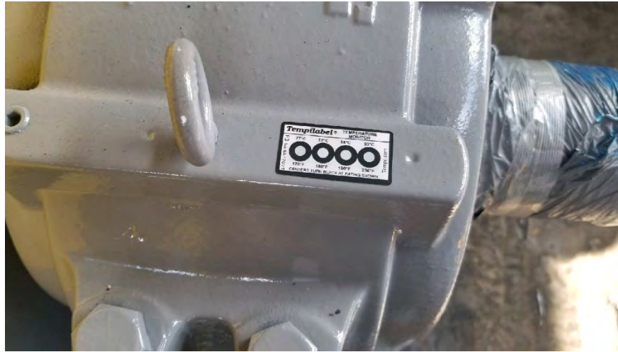
Figure 4.94: Tempilabel Temperature Monitoring Decal
