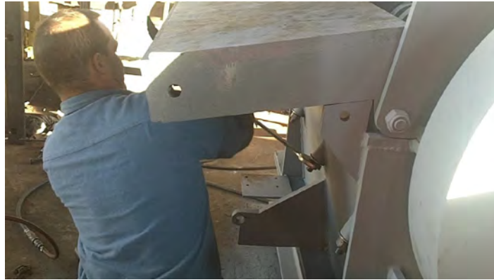
Figure 4.109: Tightening Fasteners for Screen Hold Down Bolts
