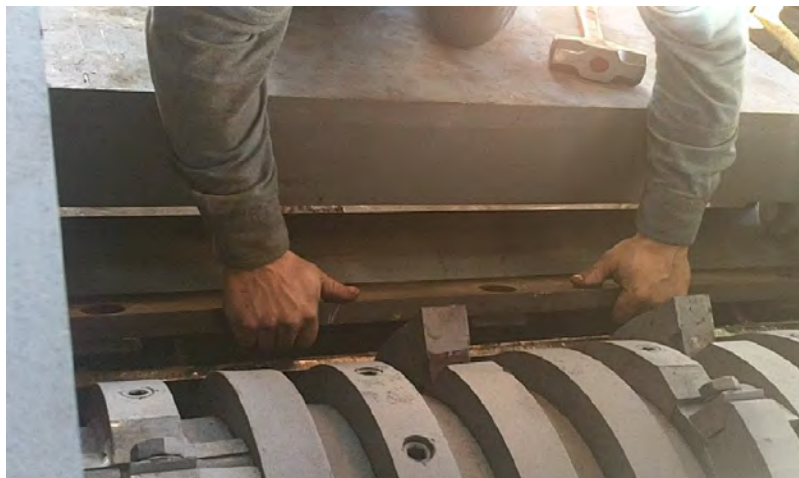
Figure 4.99: Removing Screen Clamping Bar
