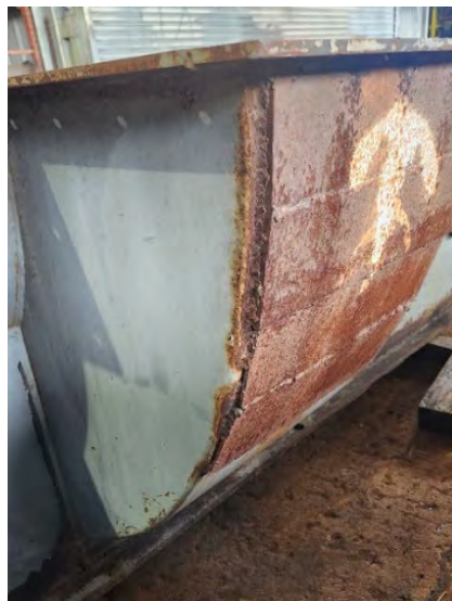
Figure 5.17: Patches to Worn Fan Scroll
